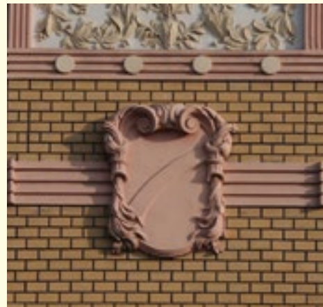
A fragment of Art Nouveau decorations on the 1905 house located at 7 Plac Ratuszowy with a motif of a cartouche, embedded in the wall faced with the clinker brick and decorated with reliefs depicting laurel leaves.
