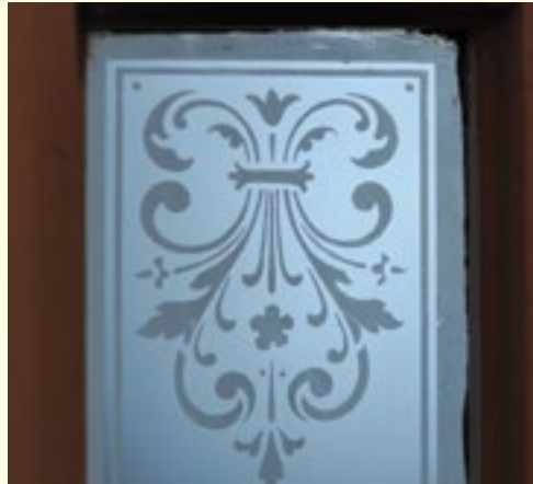
A fragment of etched decoration on the glass infill of the door in Karl Wenzel's villa at 26 Krasieńskiego Street. The surface of the pattern remains transparent and contrasts with the mat background of the glass pane.
