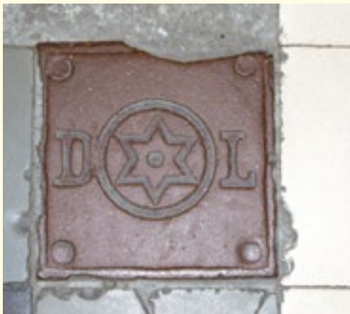
A floor tile in Johann Sabella's residential house at 19 Mickiewicza Street dating back to 1881, designed by Karl Korn. Although associated with Jewish symbolism, the pattern on the tile depicts the trademark of the ceramic products manufacturer "Dziewulski and Lange" from Opoczno.
