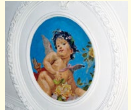
A plafond and ceiling stuccowork adorning the hall of former Eduard Zipser's villa at 52 Bystrzańska Street.
