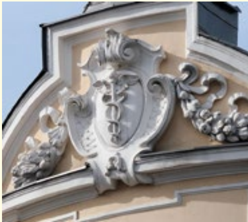
The attic in a residential house of David Feiner, a merchant. The building has stood at 1 Plac Wolności since 1902. The Asclepius wand depicted on the cartouche refers to the oldest pharmacy in Biała named „Pod Białym Orłem” [“Under the White Eagle”] that used to stand in this place.
