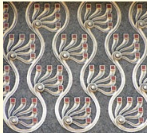
A fragment of decorative elements adorning the Jakubeckis' residential house dating back to 1903, standing between 51 Stojalowskiego Street and Głęboka Street, designed by Leopold Bauer. Mosaic squares complement Art Nouveau flowing lines.
