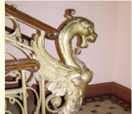
A cast iron griffin ending the forged stair balustrade, fitted at the bottom of the staircase in a villa of Emanuel Rost, Jr., located at 48 Komorowicka Street. It guarded the entrance to many residential houses and was used as a handle.
