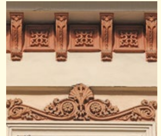
Stuccowork adorning the house at No. 25, 11 Listopada Street, originating from the end of the 18th century. Decorations on the façade, window cornices and a frieze under the eaves, however, are newer and originate from the time of restoration in ca. 1860.
