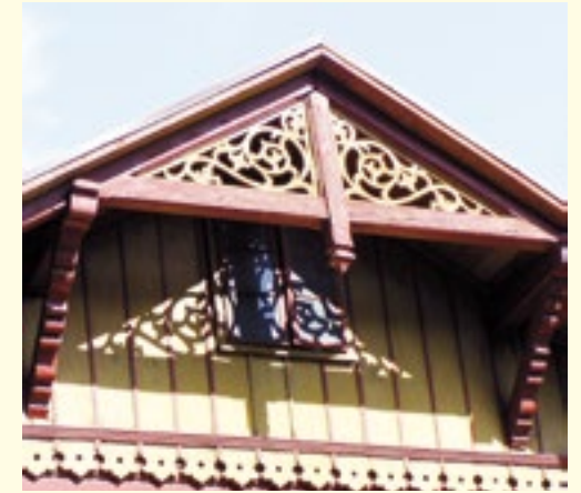
Gable decoration in Maria Hähnel's villa dating back to the 80s of the 19th century, situated in Cygański Las [Gypsy Forest] at 77 Olszówka Street. Ornate lacy wood carvings adorn the first floor and the veranda of the building.
